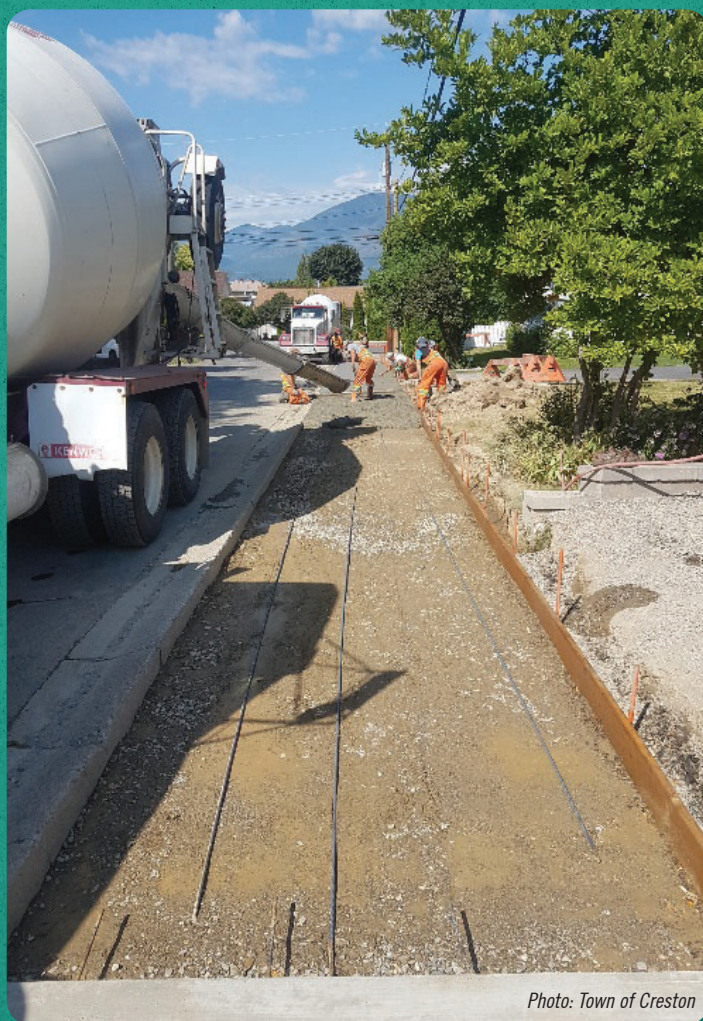
Installation of new sidewalk on Cedar Street
